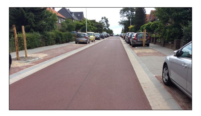
**Preventing doorings is a safety priority.** Street designs that move parked cars off the road and incorporate buffer zone next to the parking area will help keep cyclists towards the centre of the roadway, providing plenty of lateral space to avoid this incident type altogether.
