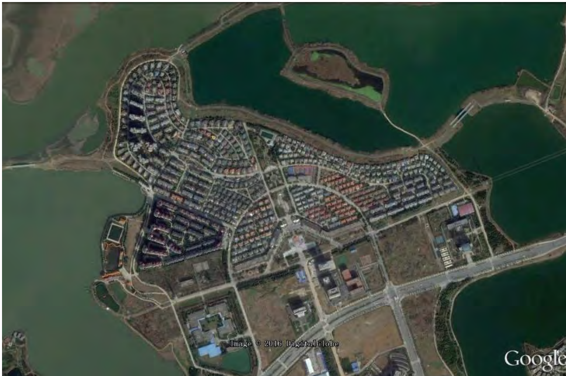
Figure 4.1.2: Villas and Low-rise Dwelling in Dongxihu's Spillover Area (Source: Google Earth, image date: 2016)
