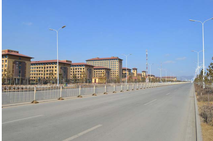
Figure 30: The campus areas are enormous and as of the Site Visit, mostly uninhabited.
