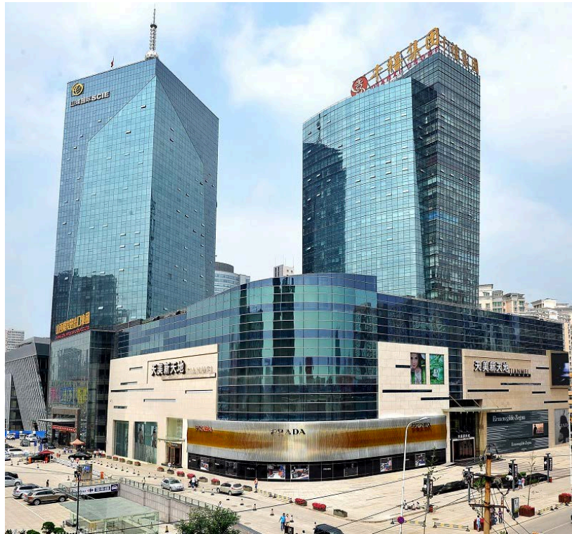
Figure 77: Tianmei Xintiandi, a new shopping and office square on the north side of Changfengjie. Directly across the street is its second half, Beimei Xintiandi. On the left, Shanxi Coal International Energy Group's headquarters.
