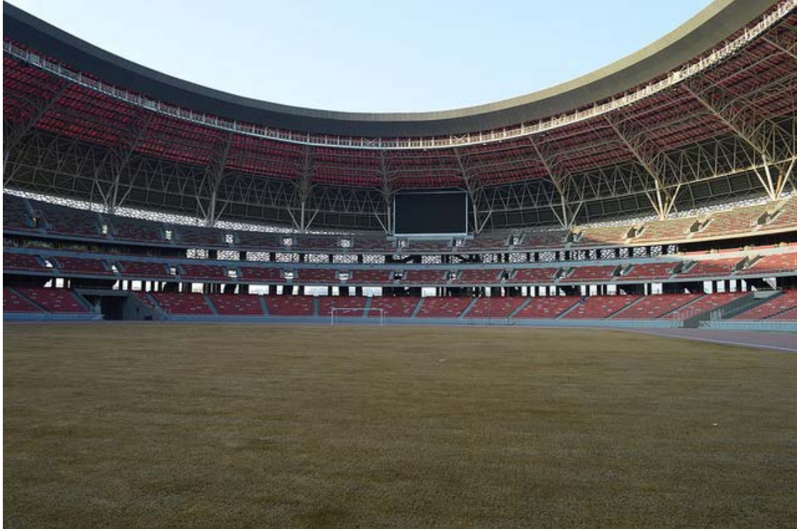
Figure 46: Red Lantern Stadium, from the pitch. The guard rail that would normally prevent fans from storming the field had been intentionally damaged, allowing access to the field- which was otherwise in very good condition. Site visit, 2014.
