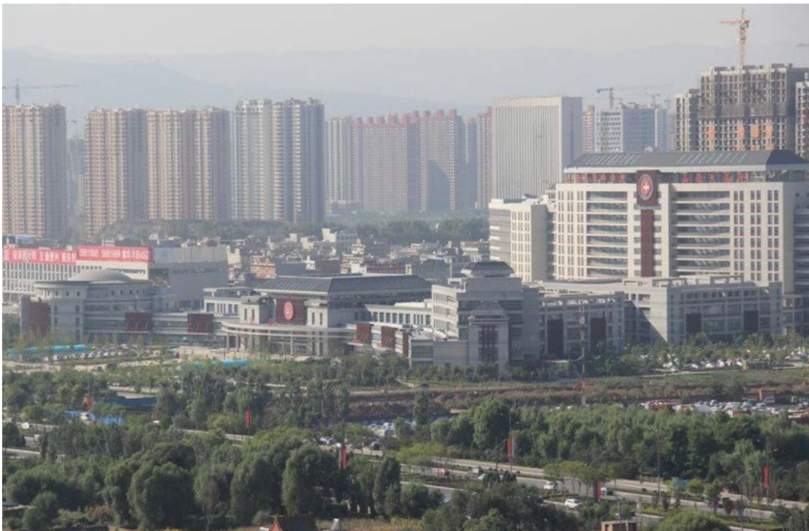
Figure 70: Shanxi Hospital. Apartments can be seen being built along the skyline.
