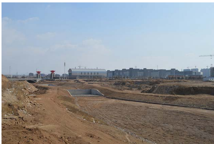
Figure 31: The digging for the University City river canal. Site Visit, 2014.
