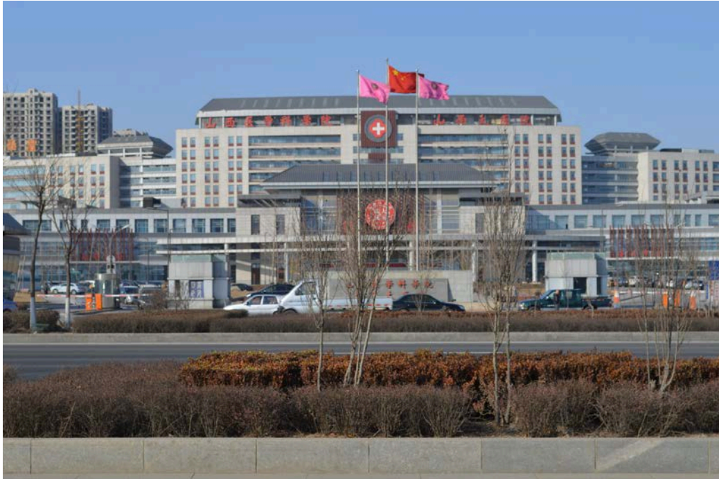
Figure 65: Shanxi Hospital, on Longcheng Road. Site Visit, 2014.
